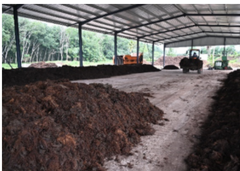
Covered composting infrastructure at the pilot site to protect compost from heavy rain and sunshine. © Jacques Fuchs, FiBL
