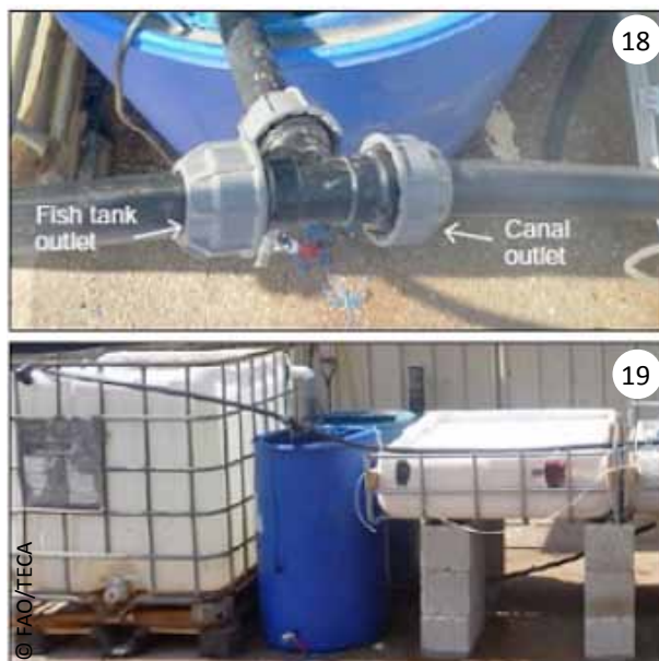
Figure 10: T-connector connecting the fish tank with the canal
