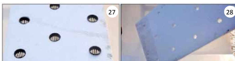
Figure 14: Polystyrene cutting and placement
