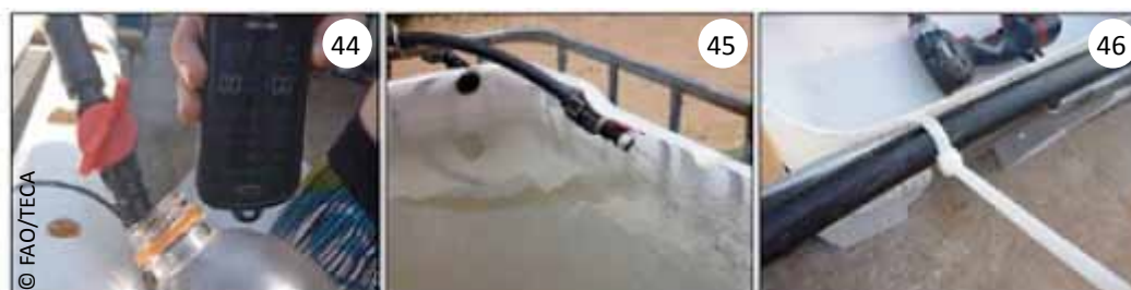
Figure 17: Secure pipes with plastic cable
