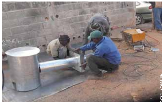
Figure 3: Smoke generator system
